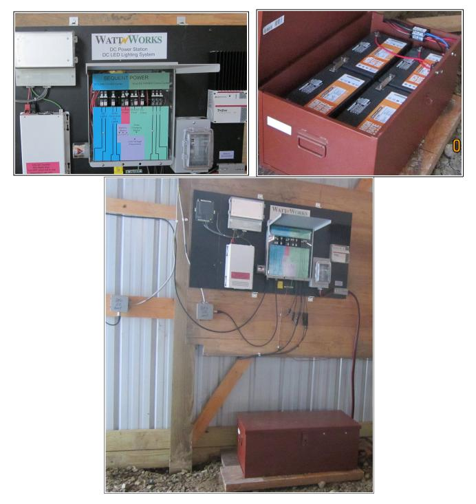
Basic DCLP Power Station 500 watts PV Panels & Racking solutions 2 - LED Wall Packs, 2 - LED Indoor Low Bays Battery Bank 2400 Watt-hours (4800 option) Minimal Optional DC Loads Large DCLP Power Station 1500 Watts PV panels 6 Wall Packs or Area /Street Lights 6 to 8 Indoor Lights Major Optional DC Loads Battery Bank 10000+ Watt-hours
